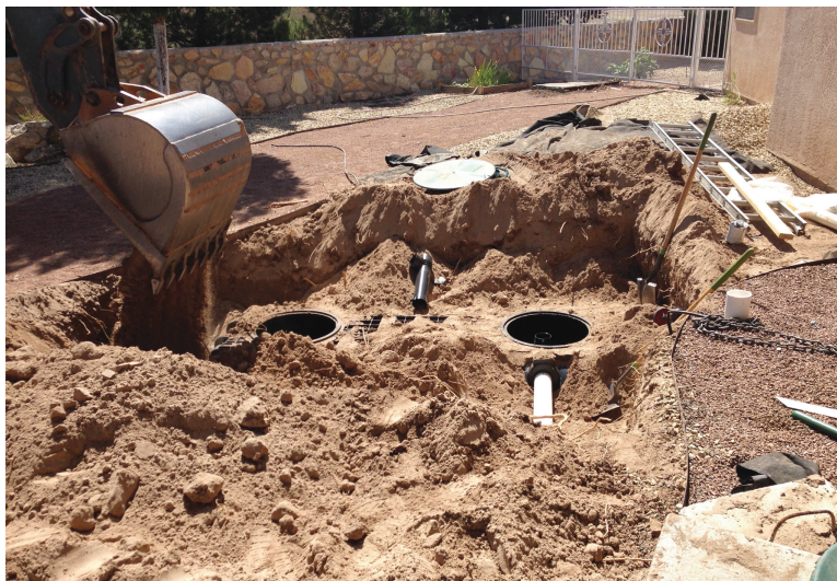
Figure 1. A septic tank being buried in a yard.
