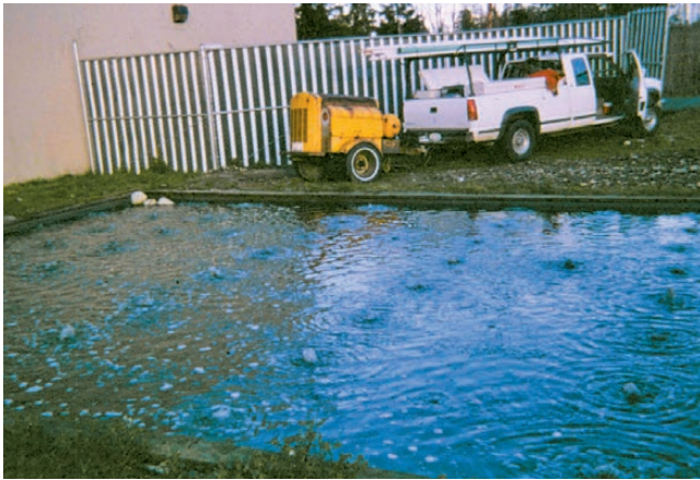
Figure 4-18. Aeration system being operated using a portable compressor (CIDWT, 2008).
