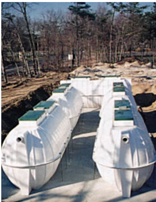
Figure 5-5. Commercially available true batch SBR system.
