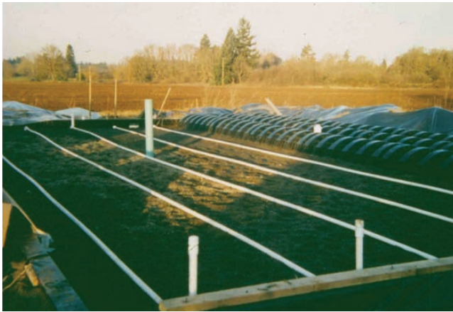
Figure 4-16. High-strength waste RSF/RGF influent distribution system (CIDWT, 2008).
