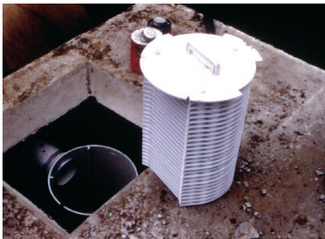
Figure 3-8. Housing for effluent screen located directly under tank opening (left). Cutaway tank showing position of effluent screen relative to attached riser (right).
