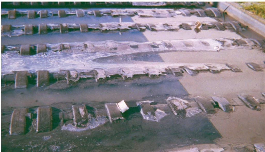
Figure 4-17. RSF damaged by wax and wax stripper discharge onto filter (CIDWT, 2008).
