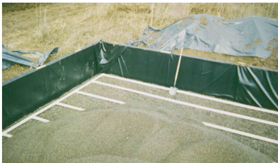
Figure 4-15. The aeration system placed below the media and above support gravel.
