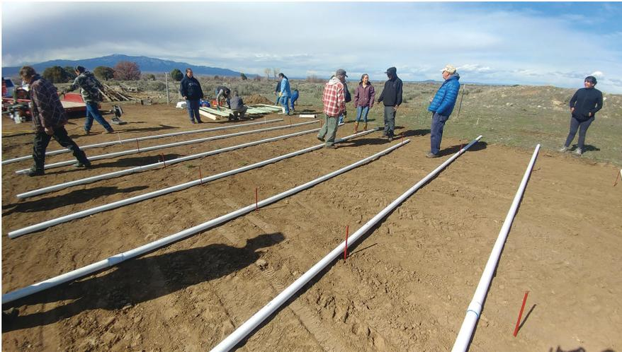
**Figure 4.** Laying out the plastic PVC pipe for the hoops for the high tunnel hoop house.
