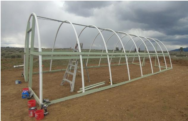
**Figure 11.** High tunnel hoop house structure.
