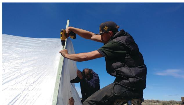
Figure 17. Use a furring strip to attach the UV protectant plastic to end wall on the high tunnel hoop house.
