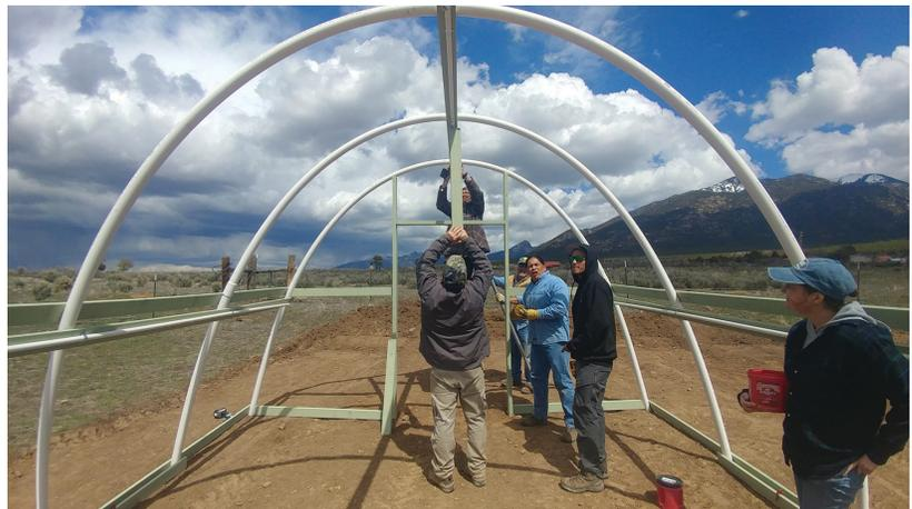
*Figure 8. Attaching 3/4-in. water pipe lines to the batten boards.*
