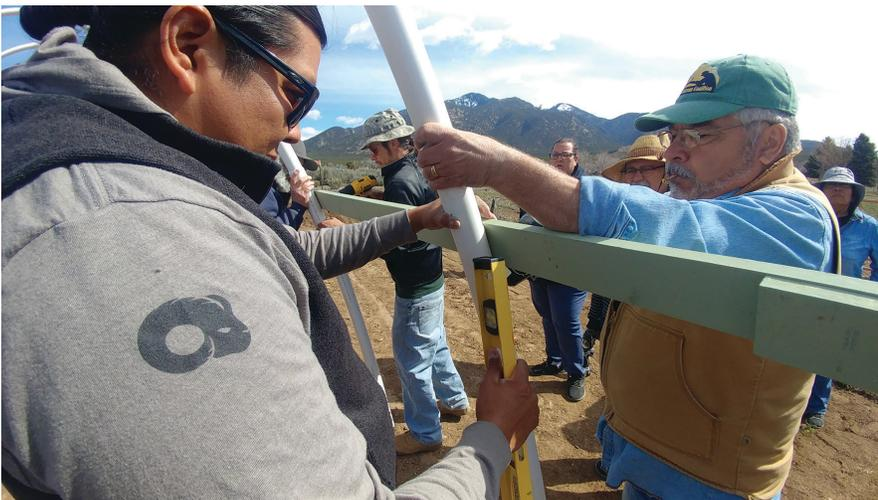
**Figure 6.** Using an I-beam level to ensure the side braces are level.
