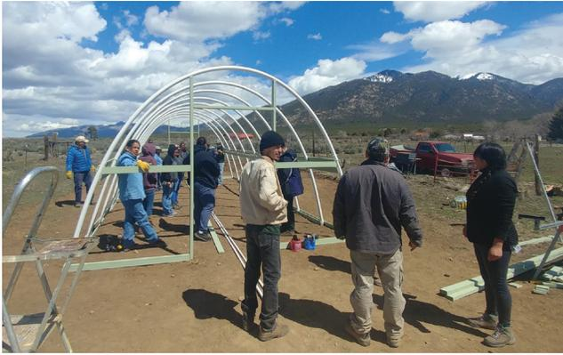
**Figure 10.** Framing of end wall on high tunnel hoop house.
