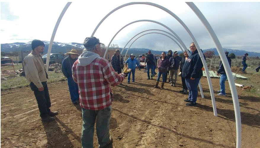
**Figure 5.** Bending the PVC pipe for the high tunnel hoop house.
