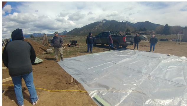
Figure 14. Laying out the UV protectant plastic cover that will cover the high tunnel hoop house.
