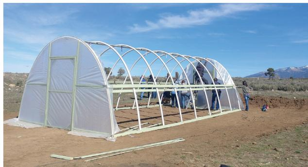
Figure 16. Attaching UV protectant plastic to the end wall on the high tunnel hoop house.
