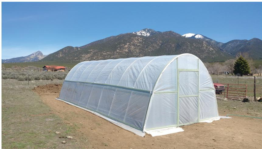
High tunnel hoop houses are a type of greenhouse structure. They are built on the ground and are large enough to walk into. For heat, they rely on passive solar heating. They are practical and economical to build.
