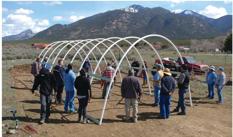
*Figure 7. High tunnel hoop house structure going up, with base and side batten boards.*
