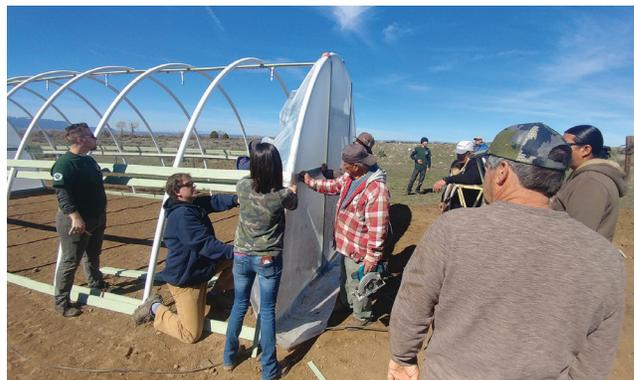
Figure 15. Attaching UV protectant plastic to the end wall on the high tunnel hoop house.
