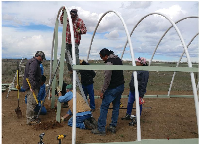
*Figure 9. Construction of end wall on high tunnel hoop house.*
