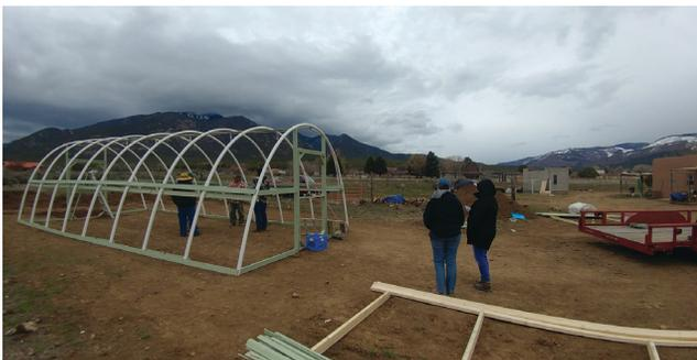
**Figure 13.** High tunnel hoop house structure with door frame installed.
