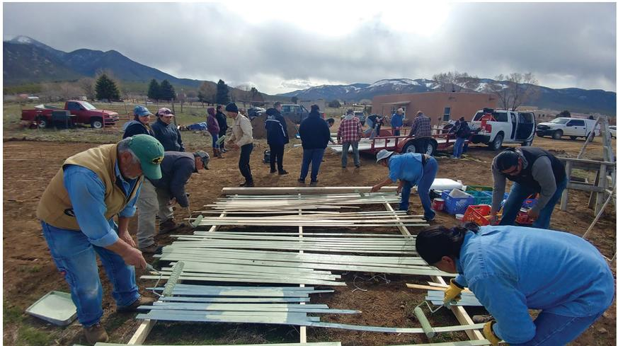
*Figure 2. Painting all wooden materials for a high tunnel hoop house.*
