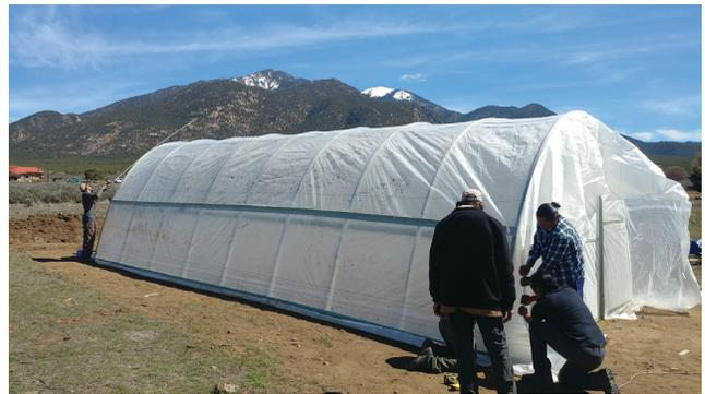
*Figure 18. Attaching UV protectant plastic over the high tunnel hoop house.*
