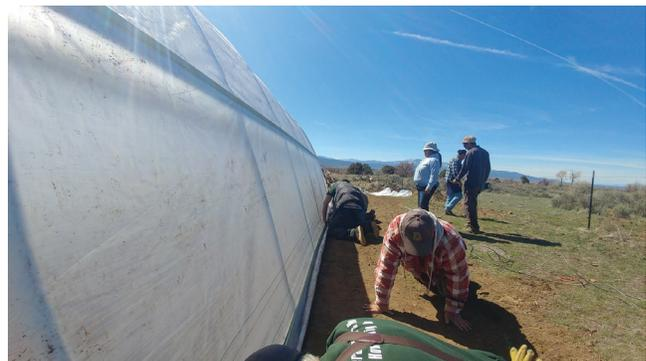
*Figure 19. Attaching UV protectant plastic to the high tunnel hoop house baseboards.*
