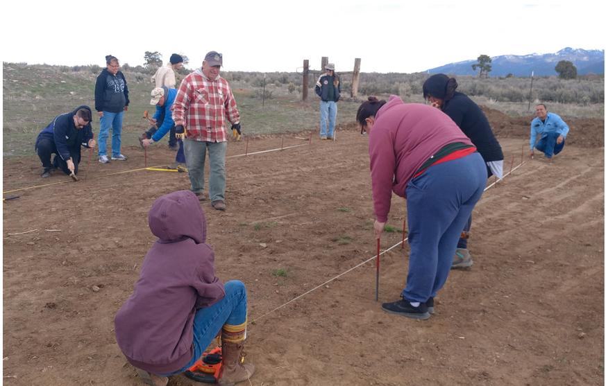
*Figure 3. Placing the rebar stakes and marking the outline of the hoop house.*
